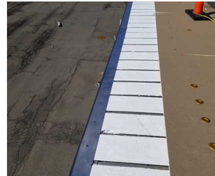
Eliminailer-T shown on flute-filled application featuring Seal-Tite Gutter
